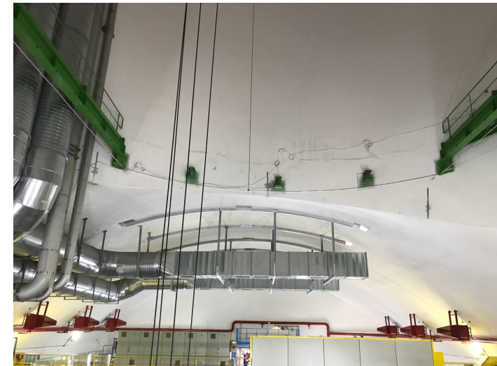
PX14 Shaft + Ceiling
