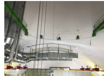
PX14 Shaft + Ceiling
