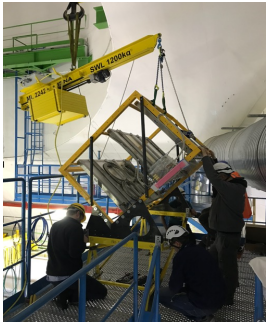
proANUBIS lowering in the ATLAS cavern
