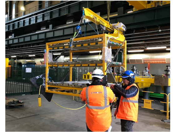
proANUBIS being lifted by Crane to pass it over through PX14 @SX15
