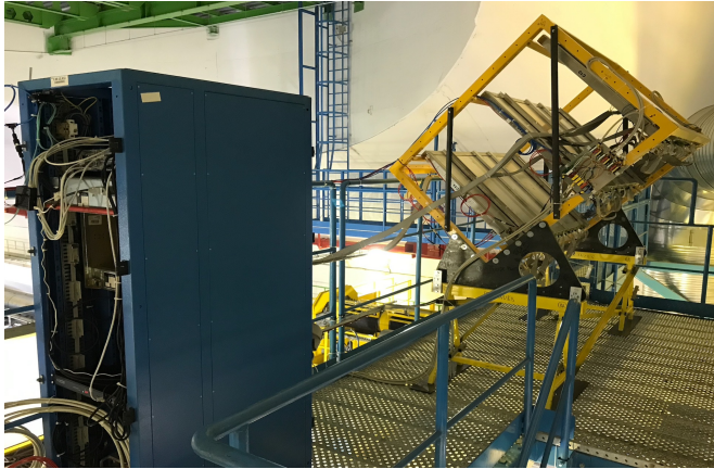
proANUBIS (DAQ + Detector) after installation
