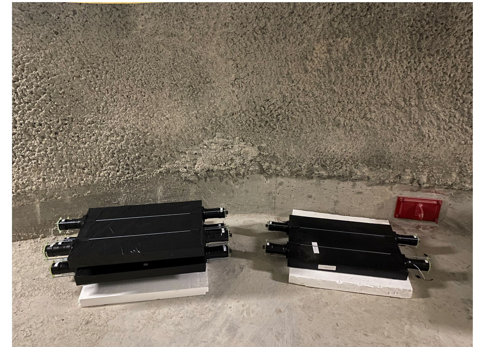
Slabs ready for installation
